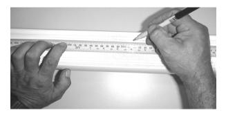
3. Determine the best positions for the wall brackets, allowing that in Gyprock or in low strength walls the brackets will be screwed into a timber stud. In more solid walls, such as masonry, position the brackets approx 150mm in from the canister end. The brackets should be no more than 450mm in from each end. You must use a minimum of 3 off wood screws per bracket or 2 off Dyna-bolts, for masonry walls and you must be satisfied that the attachment is strong enough for the a safe installation.
