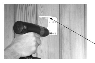
NB: Top of bracket equals top of screen canister.
