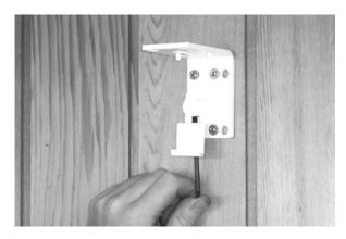
5. Using two people install the screen by placing the screen canister into the bottom of the bracket clips and pivoting back the canister to slot the top fitting rail into the T channel running along the top of the canister (you may have to remove any tape that is in the way).
