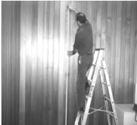
2. Measure the length of screen canister along the top surface and mark the centre of the canister with a pencil, to assist in lining up the screen when mounting.
